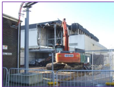
Boron Dust Plant demolition
