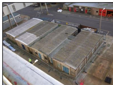
General Services Buildings demolition
