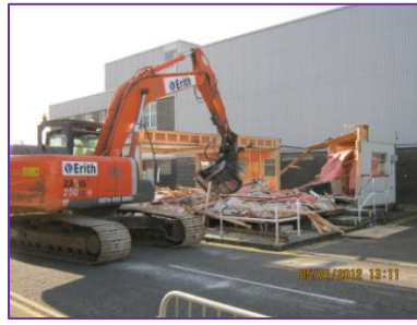
Safety Management Building demolition
