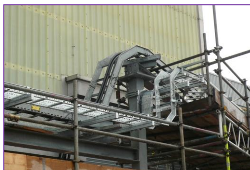
Erection of cable containment is progressing well
