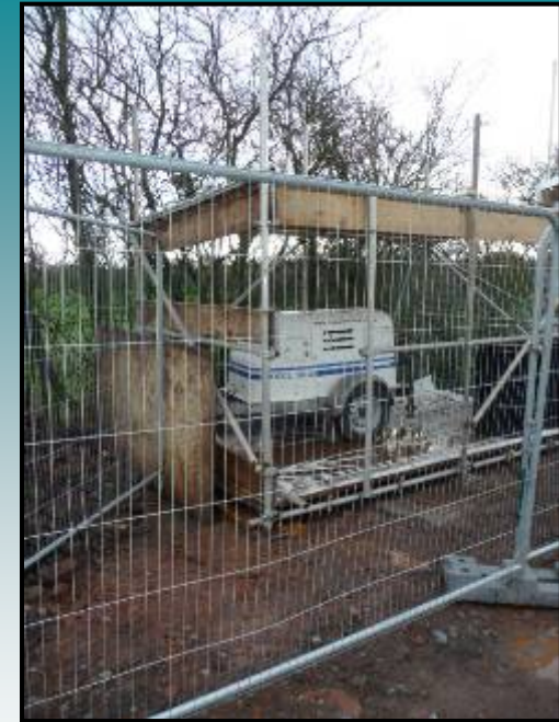
A capstan is used to assist with the pipe pulling work
